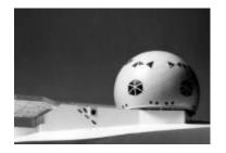
The construction conditions on the mountain's summit were subject to time restrictions due to the harsh climate, and the transport of materials was only possible through the use of cable cars and helicopters. For this reason, a geodesic dome was selected for the construction of the main building. Providing the largest possible capacity over the smallest surface, the dome promised a minimal loss of heat, as well as offering great aerodynamic and static properties. ...more...
